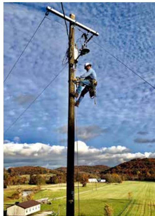
Lineman Chase Gander. Photo: Josh Hale
